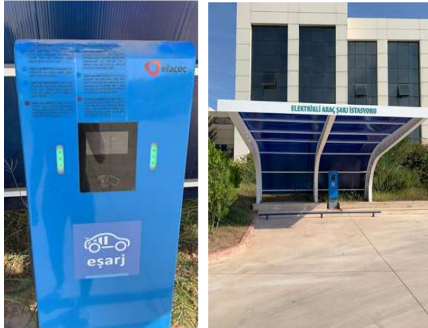
Figure 21. Charging station for electric vehicles
