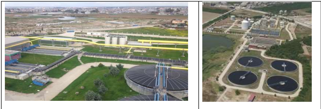
Figure 14. Yuregir Wastewater Treatment Plant
