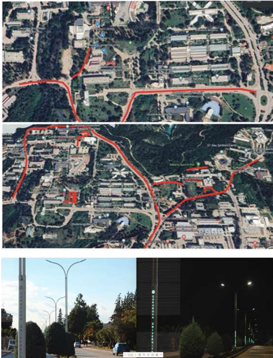
Figure 6. Settlement Plan of LED street lighting installed in 2022 and LED Street Lighting
