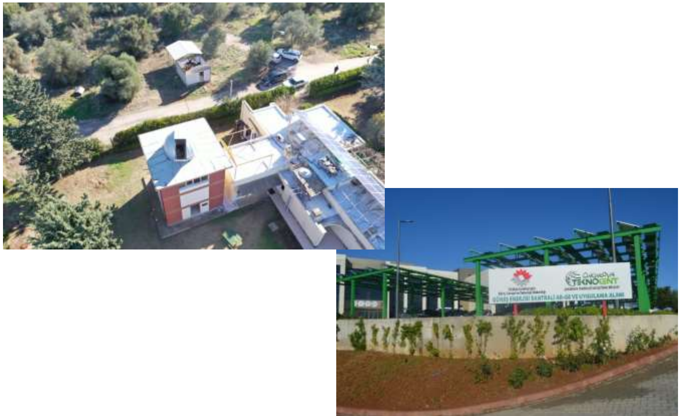
Figure 7 . PV Power Plant (Solar House and Technopark)
