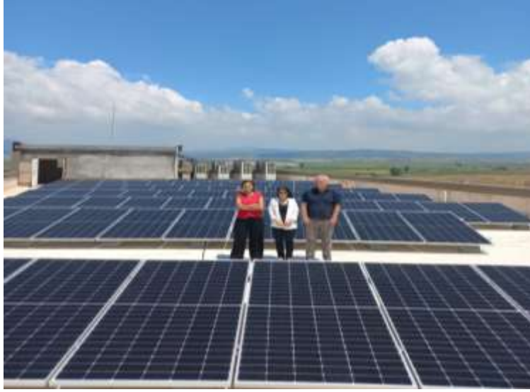
Figure 8 . Yumurtalık Vocational School Solar Power Plant
